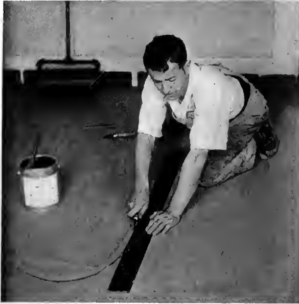
CUTTING JOINTS AND MATCHING SEAMS
